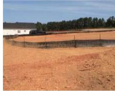
**DESCRIPTION:** Silt fence consisting of geotextile fabric stretched across steel or wood posts is required when there is any site disturbance. The lower edge of the fence is vertically trenched into the ground and covered by compacted backfill. Fencing is placed along front, side and rear property lines allowing for construction entrance.
