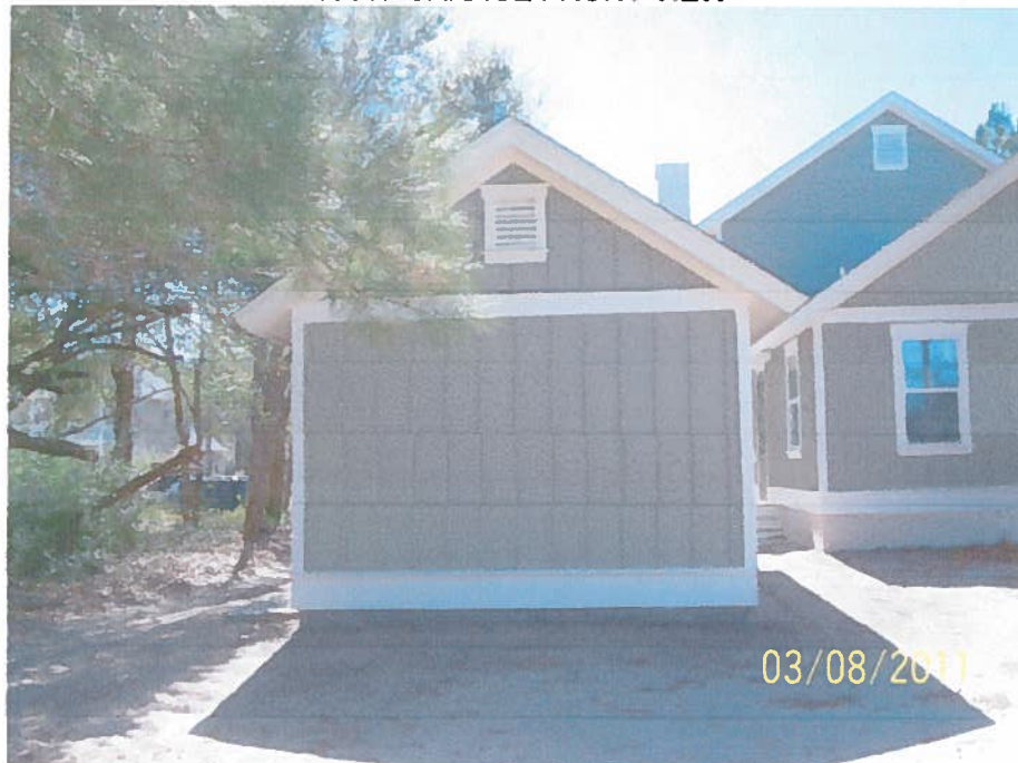
38017 REAR GARAGE VIEW
